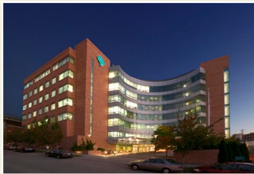
Seattle Cancer Care Alliance (SCCA) building entrance at dusk.
